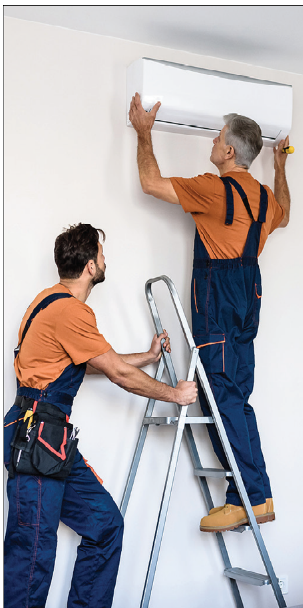
Heat pump being installed. Photo credit: BigStock
